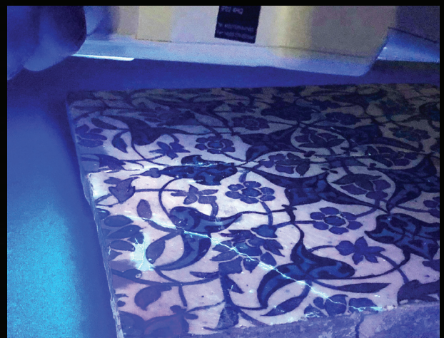
The tile after retouching with paint and matched the surrounding surface area.
