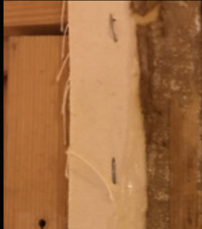
Fig. 10: Strip-lining, tacking margins)
